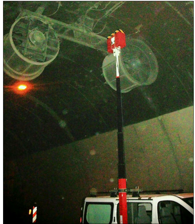
2. Tunnel lining can be quickly inspected with a retracting mast installed on a vehicle.
